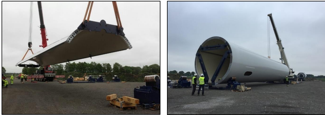
Figure 4.2.1. Multi-segment WPP mast section (Vestas LDST 27 )
