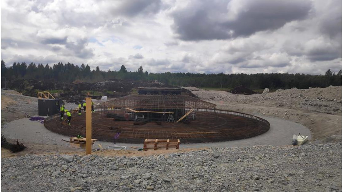
Figure 4.3.7. Part of the WPP foundation steelwork under construction (photo: Enviropojekts)
