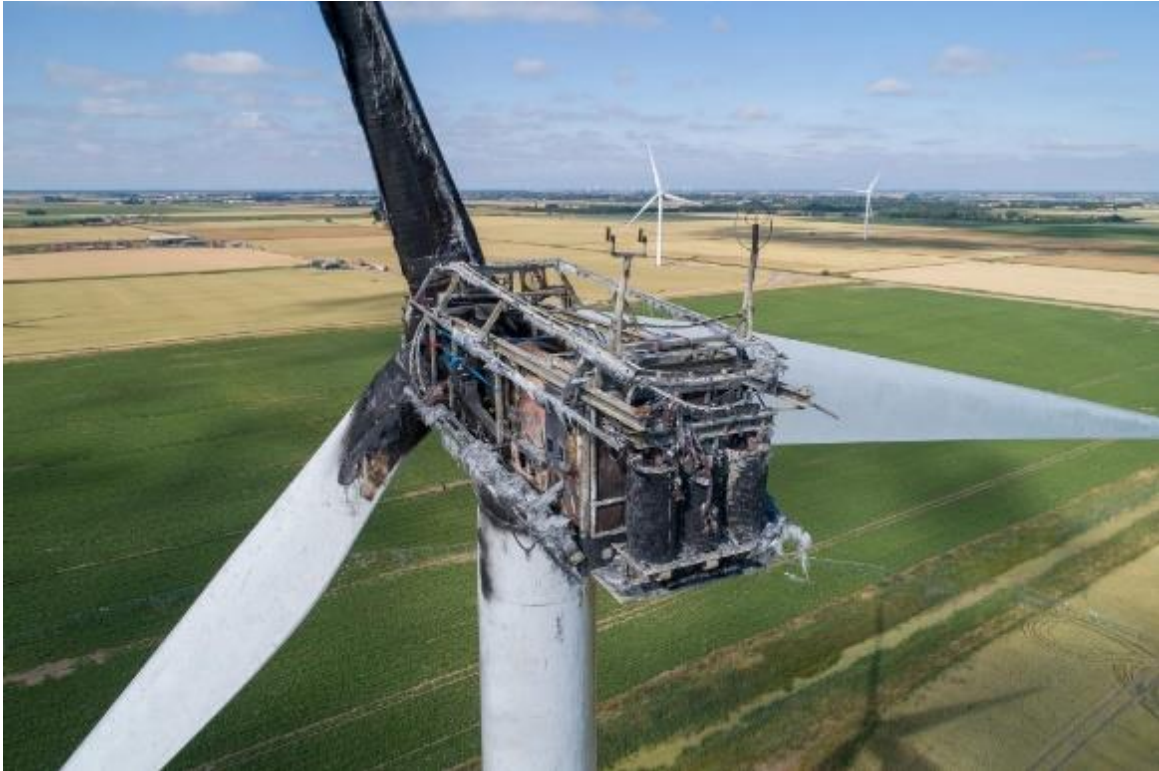
Figure 5.3.9. Damage to WPP caused by fire 80
