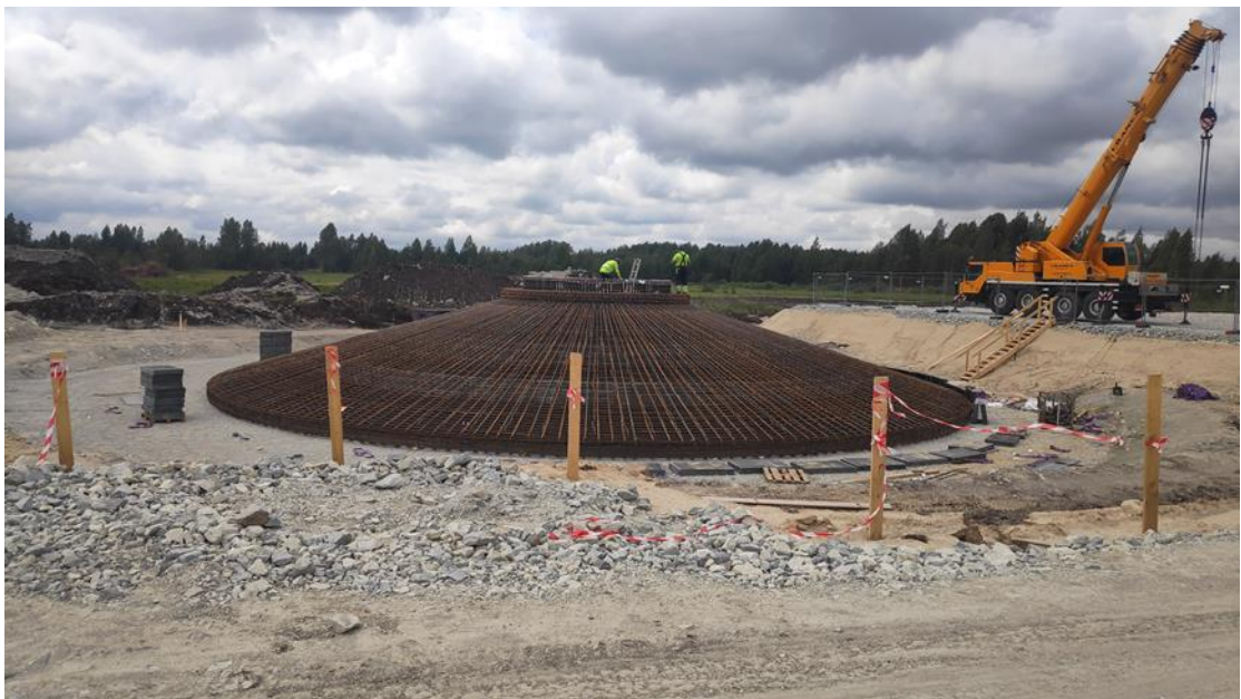
Figure 4.3.8. Part of the WPP foundation steelwork under construction (photo: Enviropojekts)
