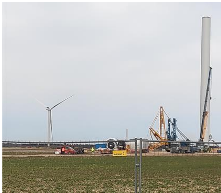
Figure 4.3.10. Installation process of a WPP turbine in Latvia - Tārgale project, 2022 (photo: Enviroprojekts)
